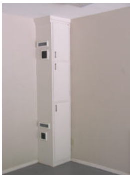
Figure 27. Equipment cabinet containing disconnect panel, UPS, DC power supply, emergency power battery, DSL modem and router. Disconnect panel is the station single point ground which connects to a power line bonded ground rod by way of the 4" aluminum strap seen at the left side of the cabinet.
