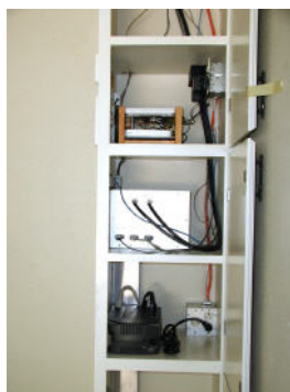
Figure 27. Equipment cabinet containing disconnect panel, UPS, DC power supply, emergency power battery, DSL modem and router. Disconnect panel is the station single point ground which connects to a power line bonded ground rod by way of the 4" aluminum strap seen at the left side of the cabinet.
