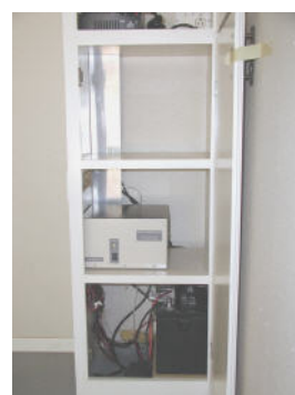
Figure 27. Equipment cabinet containing disconnect panel, UPS, DC power supply, emergency power battery, DSL modem and router. Disconnect panel is the station single point ground which connects to a power line bonded ground rod by way of the 4" aluminum strap seen at the left side of the cabinet.
